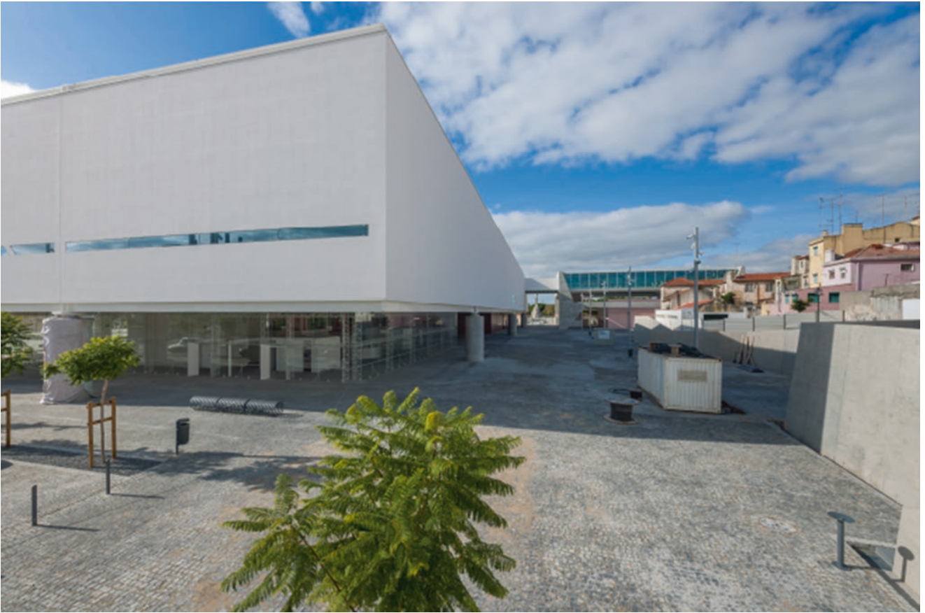
Coach Museum External view from the interior of the courtyard Copyright Arménio Teixeira
