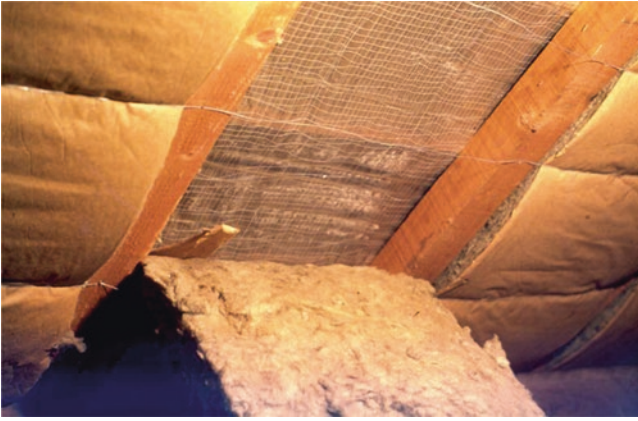
Fig. 5 Insulated pitched roofs, leaky vapour retarder and vapour-tight, non-capillary underlay. The result is an interstitial condensation deposit with run-off and water leakage at the roof edges
