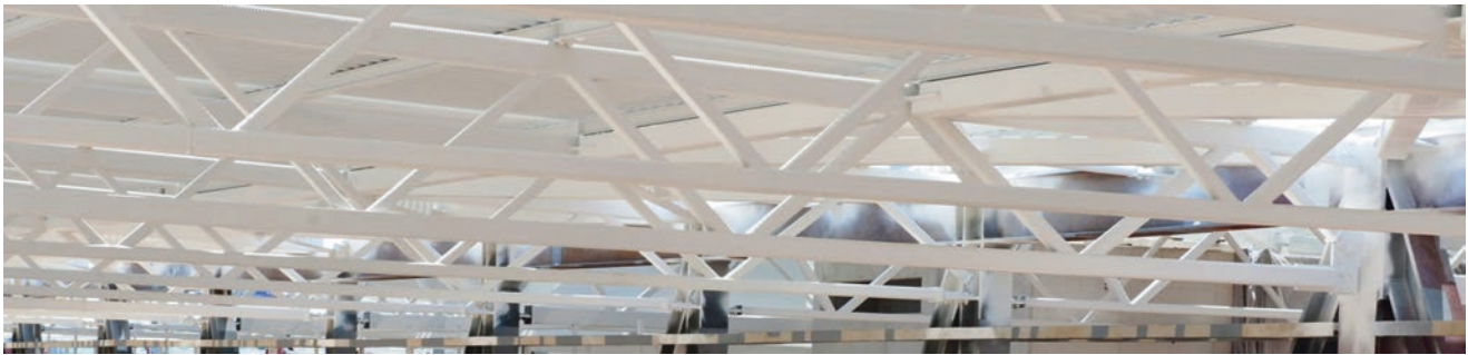
Fig. 11 Roof structure under construction
