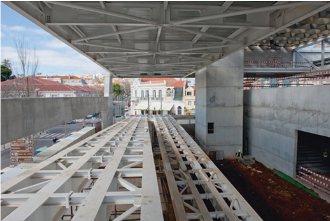
Fig. 8 Ramp under construction
