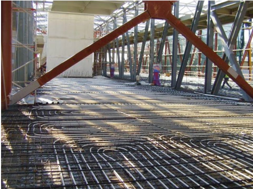
Fig. 88 Floor heating system
