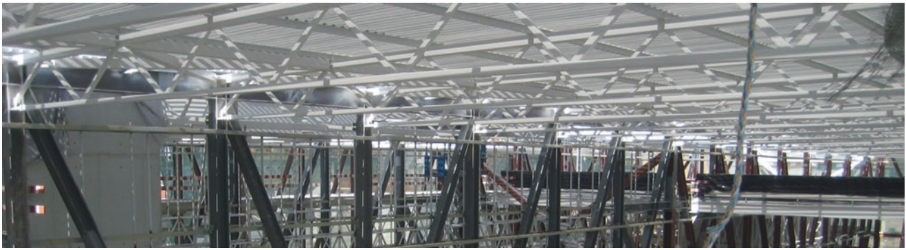
Fig. 28 Roof structure under construction
