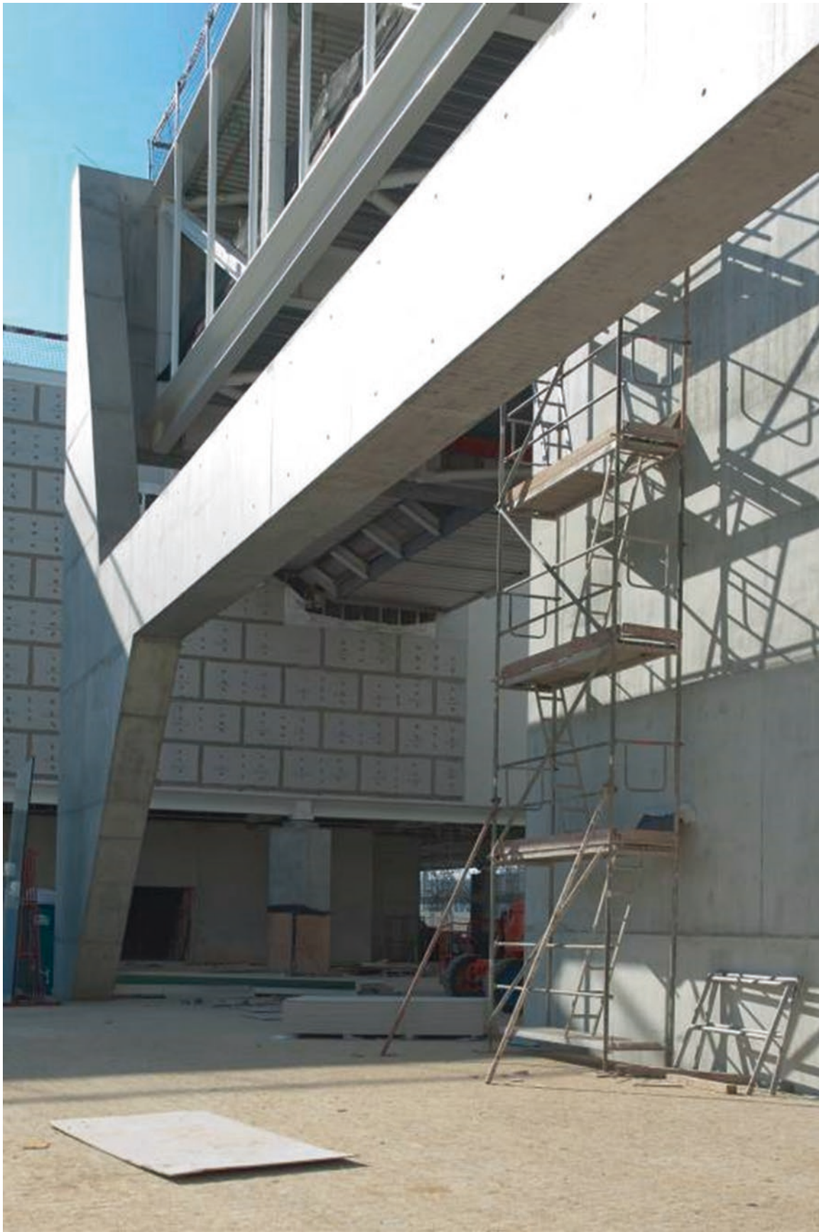
Fig. 52 Auditorium under construction before the finishing phase
