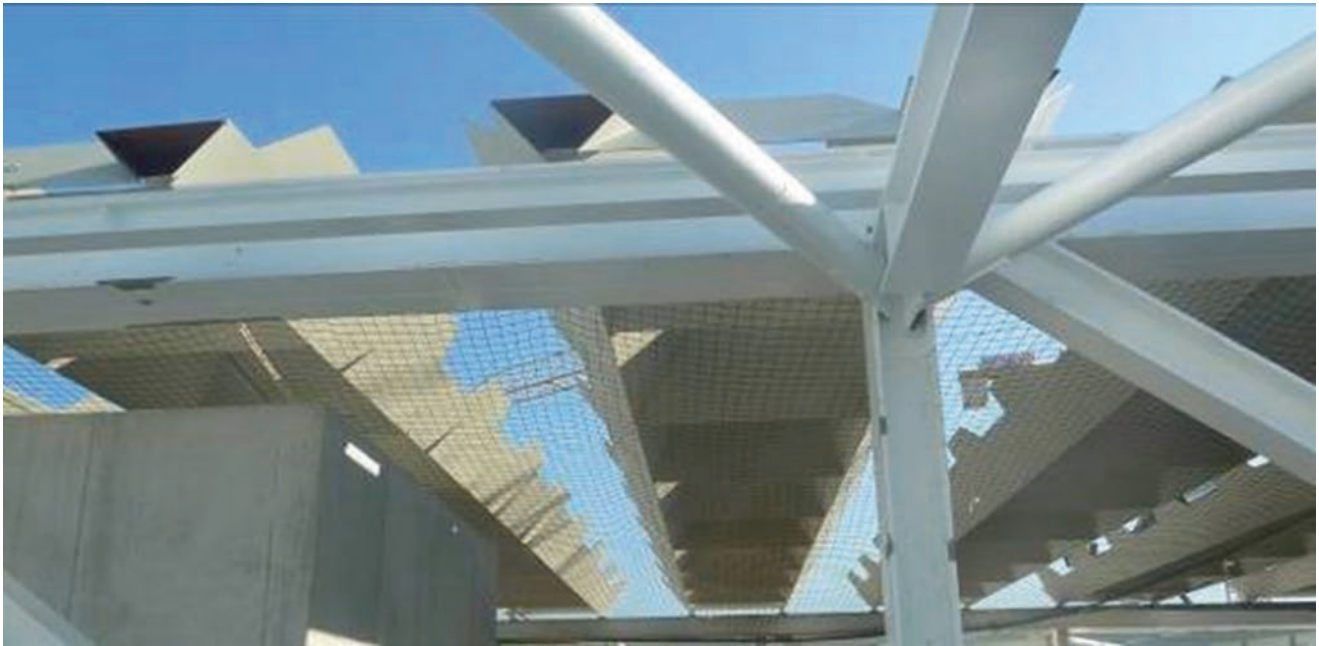
Fig. 57 Auditorium's skylight in position before assembly
