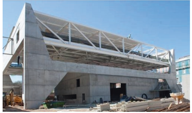
Fig. 18 Auditorium under structural construction phase
