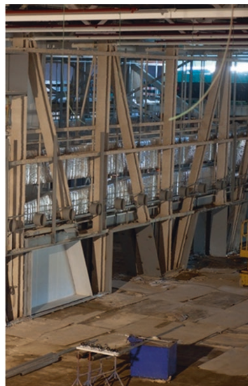
Fig. 5 Main structure of the museum during the construction from the inside
