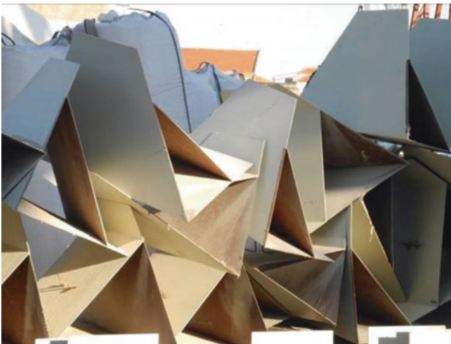
Fig. 58 Auditorium's skylight before assembly
