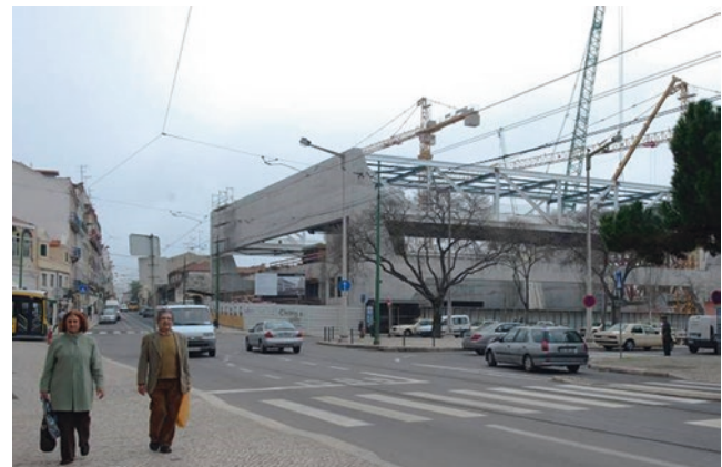
Fig. 22 Street view of the auditorium from Junqueira Street under structural construction phase
