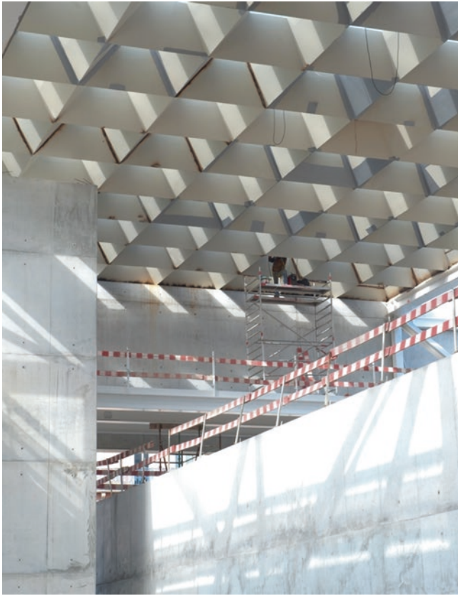
Fig. 17 Skylights of the auditorium under construction
