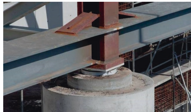
Fig. 26 Detail of the structural support of the main building's external wall under construction
