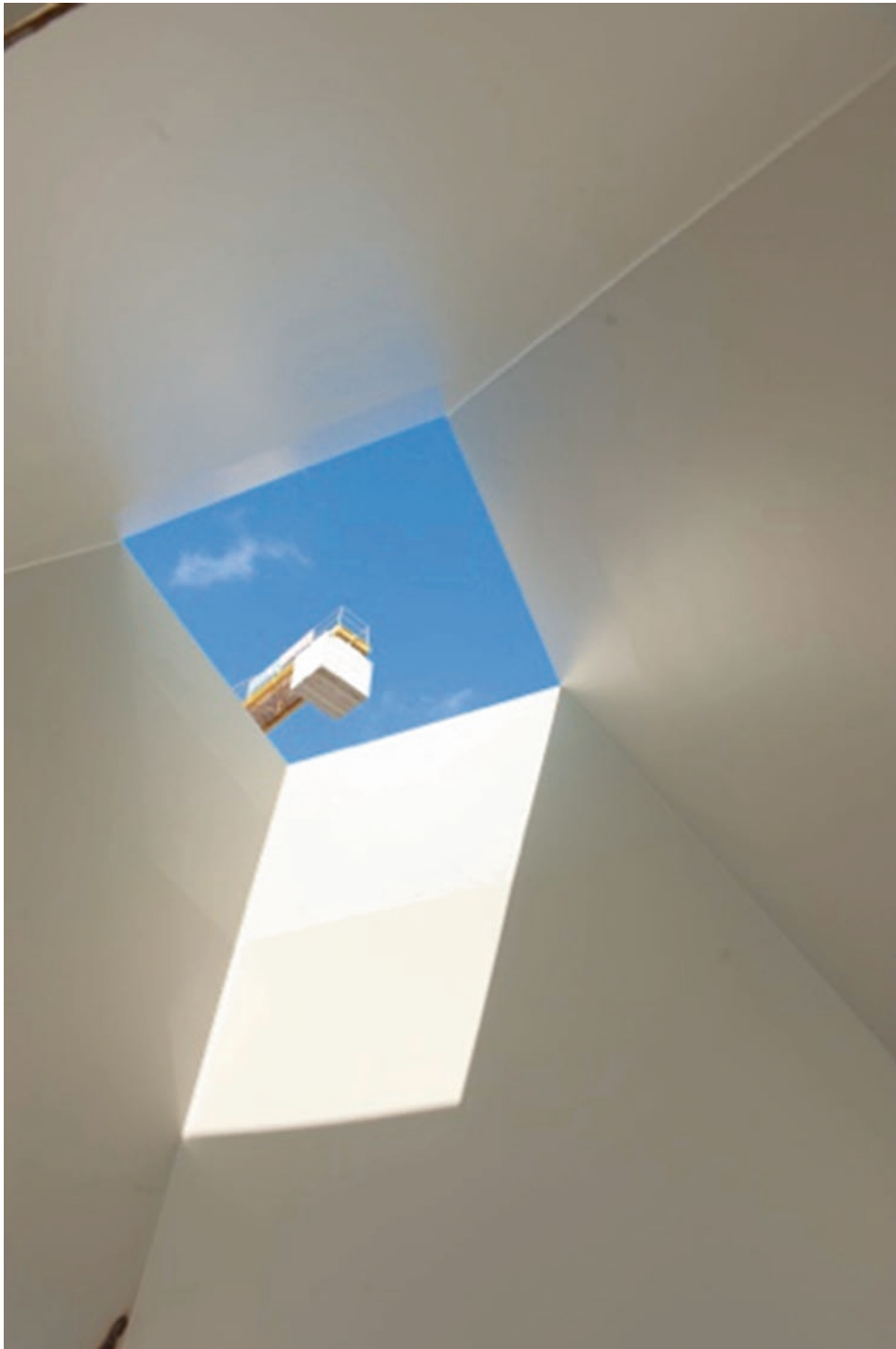
Fig. 64 Auditorium skylight's under construction
