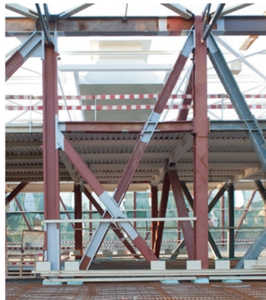
Fig. 40 Main building's external wall module under construction
