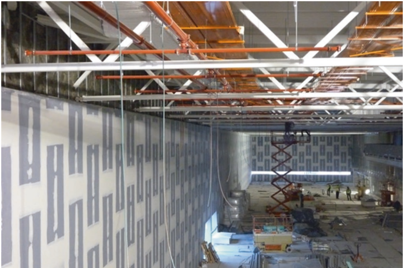
Fig. 77 Infrastructures construction phase
