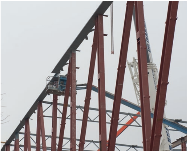
Fig. 14 Wall structure under construction
