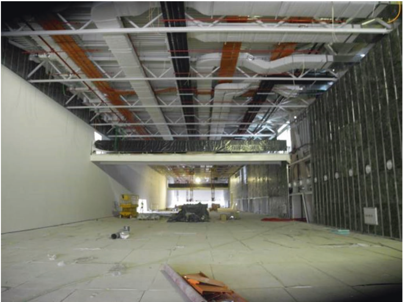
Fig. 85 Main room in the finishings construction phase
