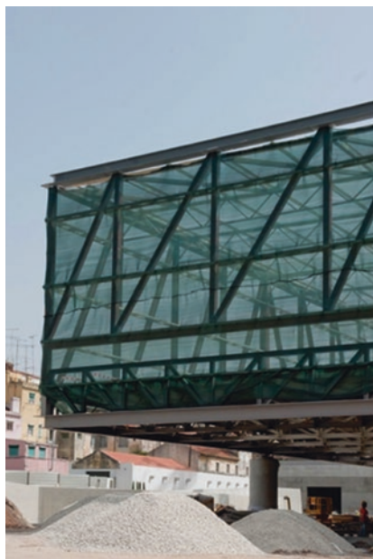
Fig. 39 Main building's external wall under construction
